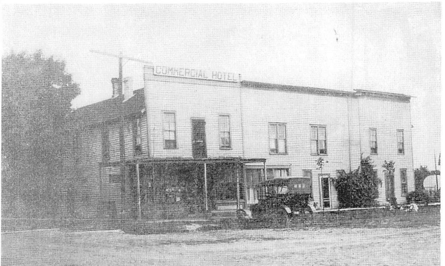
The Commercial Hotel located on the north side of east Main Street, just off First Street.
